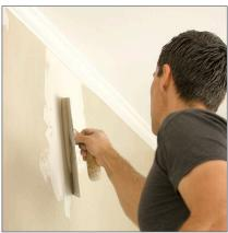
**LEFT**: Dimension Grit: Baby Bite. **RIGHT**: Baby Bite used to texturize primer going over drywall (to add grippy tooth) prior to application of a thin-coat, fine-grained interior venetian-style lime plaster finish. Also used to add subtle texture to paints and coatings.
