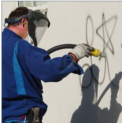
LEFT: Sand Blast Soft (SBS) grade pumice blast media. RIGHT: SBS is a smaller sand blasting grade for cleaning more delicate surfaces.
